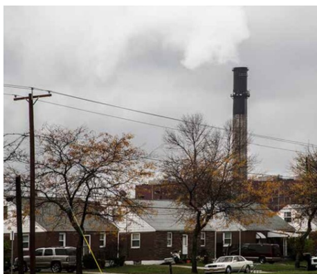
Huntley Power Station Source: IEEFA
