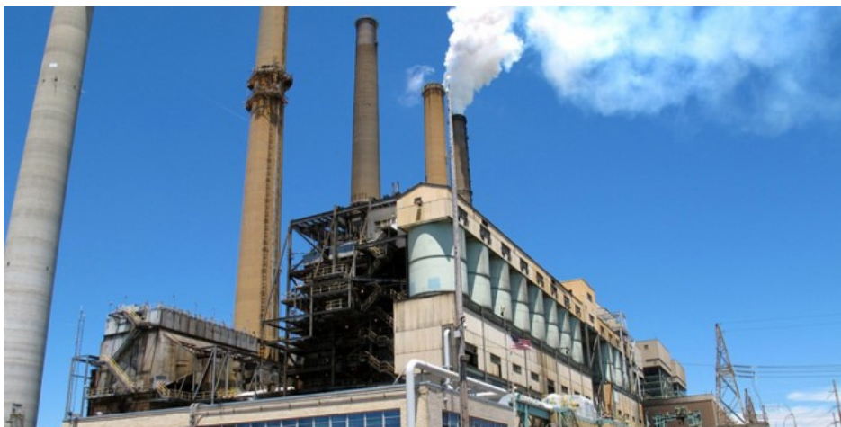
AEP's Conesville power plant
